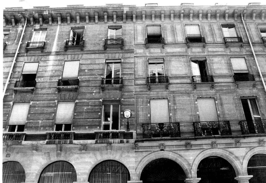
1. Building on the Chausée d'Antin, Paris. Although this is an eighteenth-century building, it nonetheless illustrates the degree to which the stone can be carved. (Unless otherwise noted, all images are by the author.)
